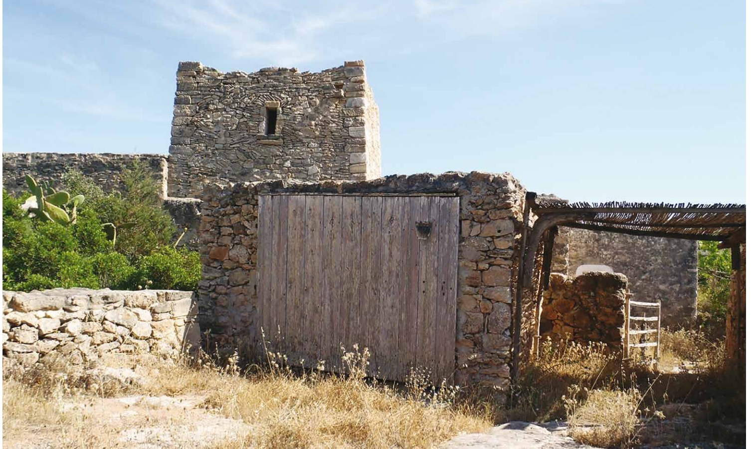
Foto: Sebastià Martorell Arquitectura tradicional, Formentera, SXIX 19 th century traditional architecture, Formentera
