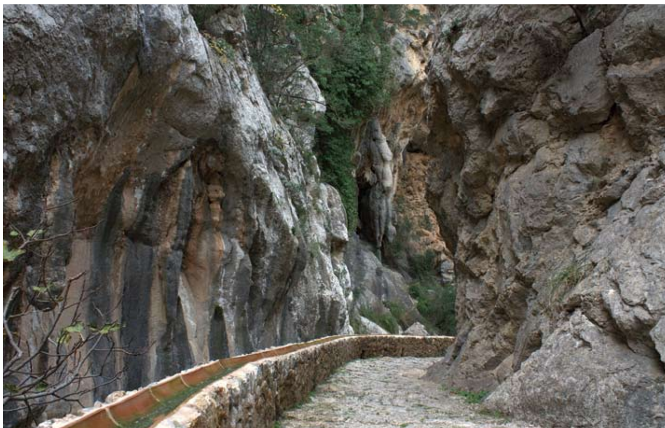
Gutter alongside the stone path (Photo: Esperança Perelló)
